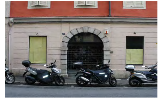
locale al piano terra
